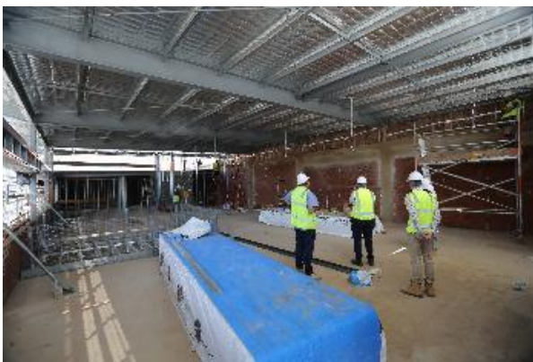
Figure 1: New roof on for 1st floor worship space
