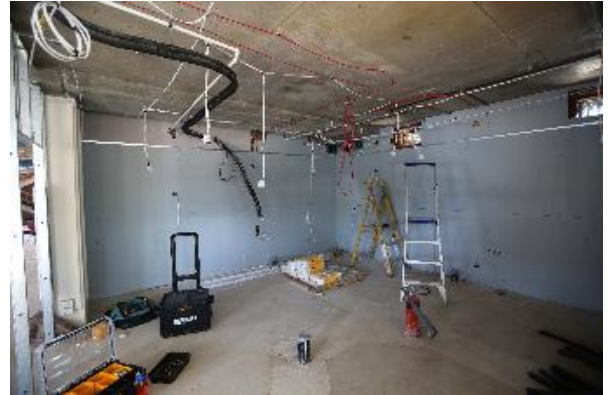
Figure 4: New ground floor accessible bathrooms
